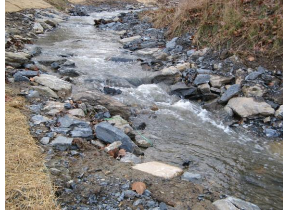
After emergency stabilization of failed reach
