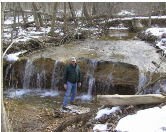
Headcut in Legacy sediments below sewerline on Feb 9, 2004
