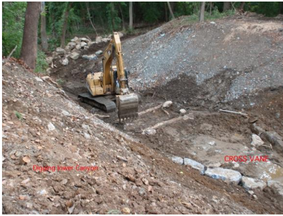
Digging the new streambed through the canyon
