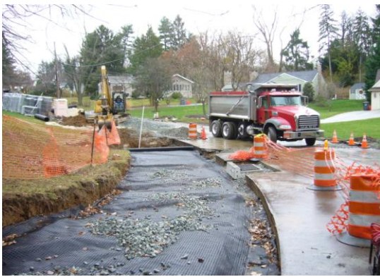
Large infiltration project above storm water outfall
