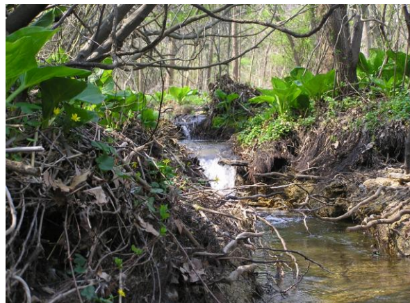
Headcuts erode the lower edge of sediment flume below RR tunnel
